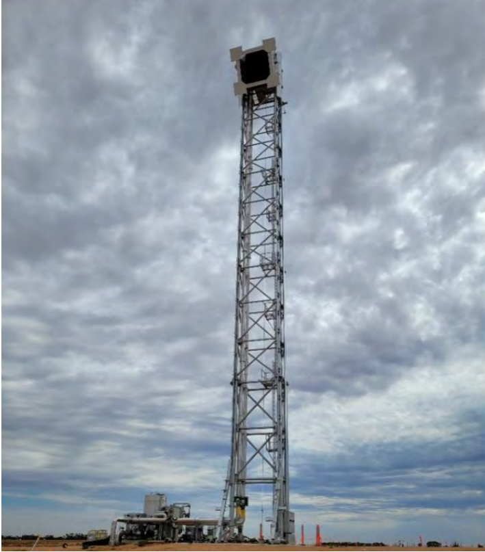
Figure 6 Receiving tower Carwarp Solar Farm
