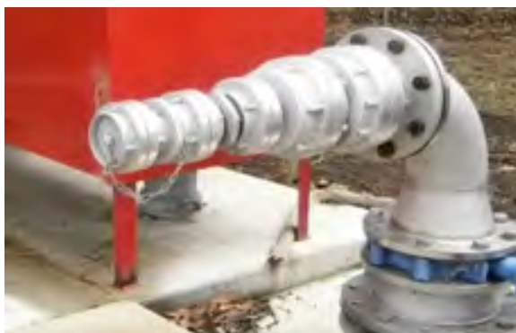
Figure 4: 125mm, 100mm, 90mm, 75mm, 65mm Storz tree adapters.
