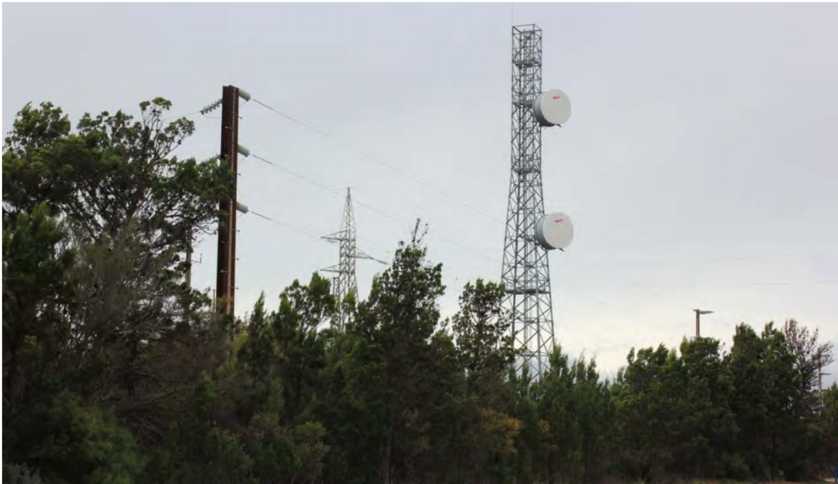
Figure 22: View of existing infrastructure associated with substation
