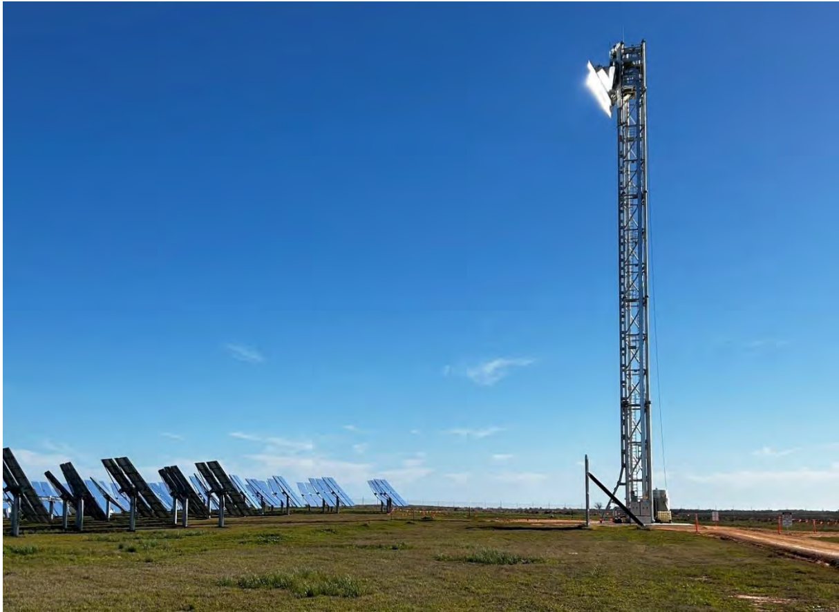
Figure 1 - Articulated mirrors (heliostats) and PV Ultra Receiver – Carwarp Victoria
