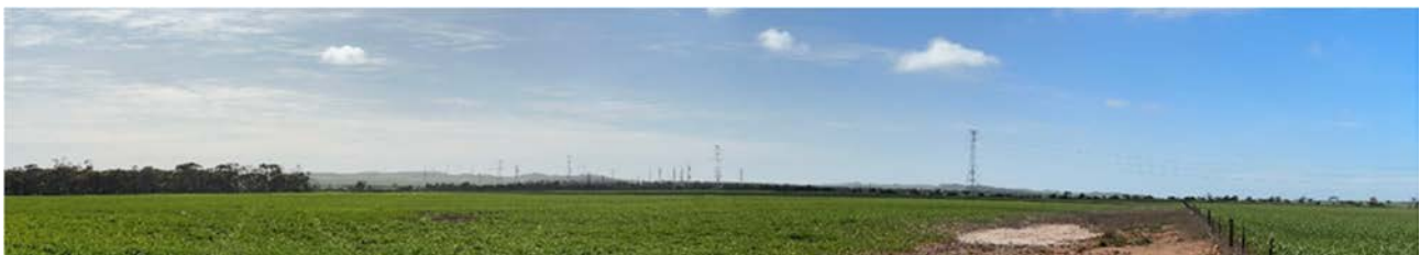
Figure 4: Transmission line with towers evident across the subject land and beyond (including Yadnarie substation). Photograph from the principal driveway to 4543 Birdseye Highway, looking in a north easterly direction.
