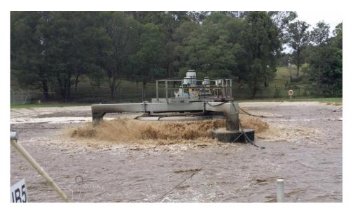
Figure 6: Mechanical surface aerator on a wastewater treatment lagoon (photo Simmonds & Bristow Jan 2016)
