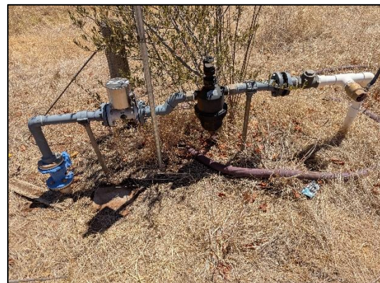
Existing Ø150mm recycled water main and Ø60mm recycled water connection owned by Barossa Infrastructure Ltd
