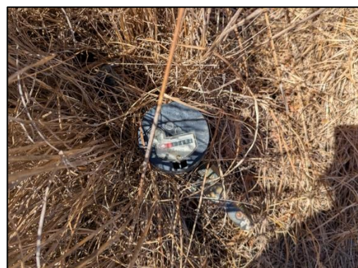
Existing Ø20mm water meter connection located on Hoffnungsthal Road (ID: M51201375)
