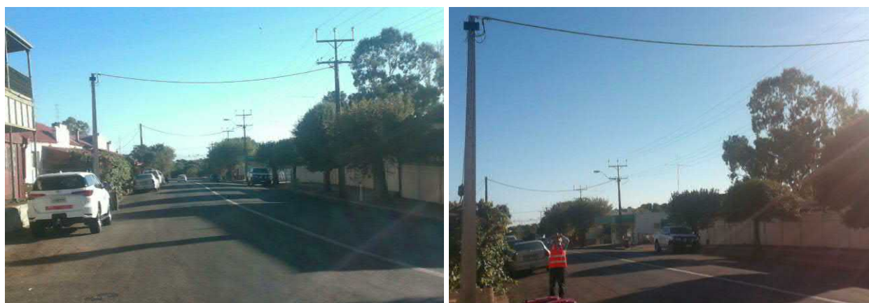
Figure 3 Existing overhead power lines on Worlds End Highway
