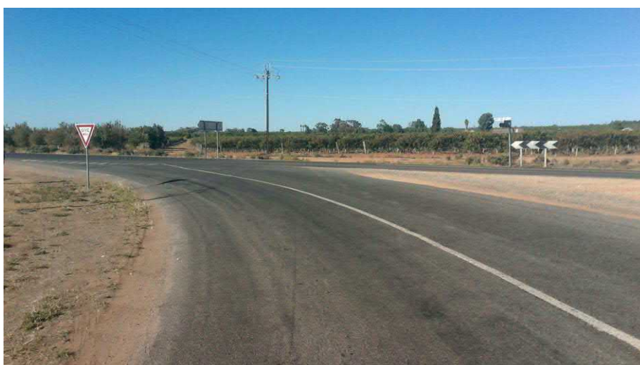
Figure 8 Low angle of entry onto Ral Ral Avenue from Wentworth Renmark Road
