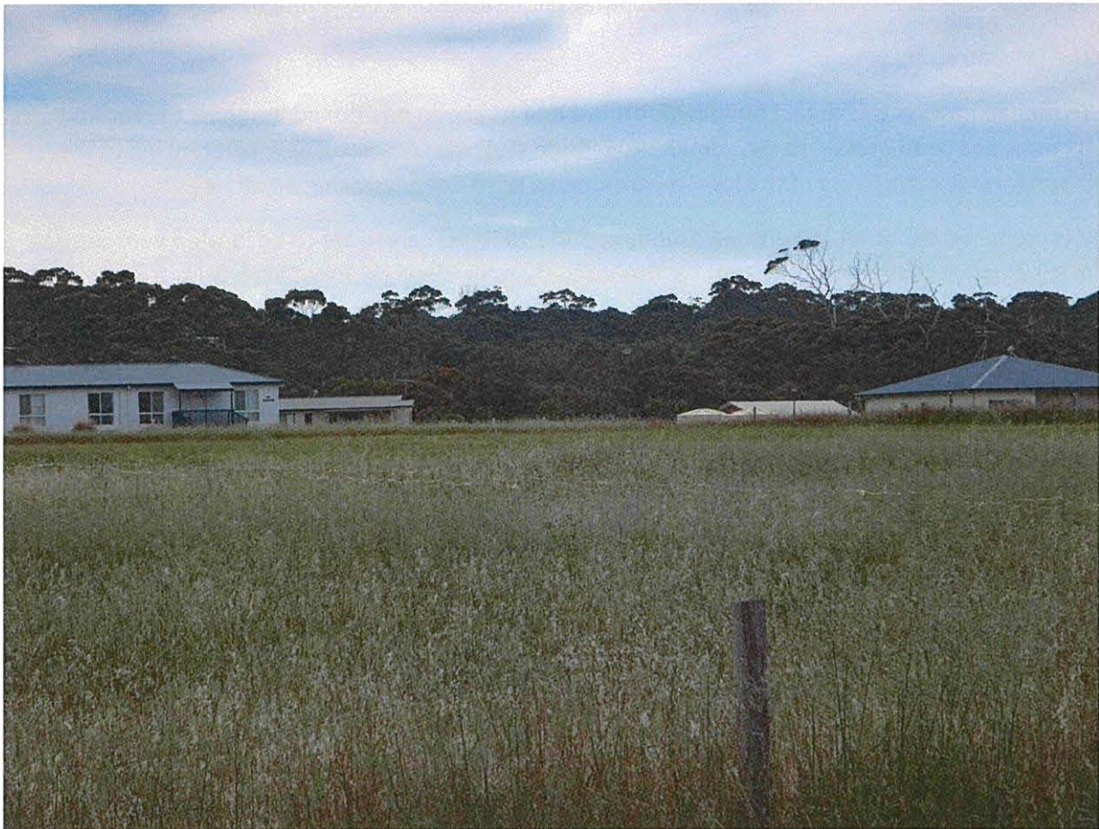
A view of the holiday shacks/residents houses and the backdrop of the proposed resort where ten six storey towers are proposed.
