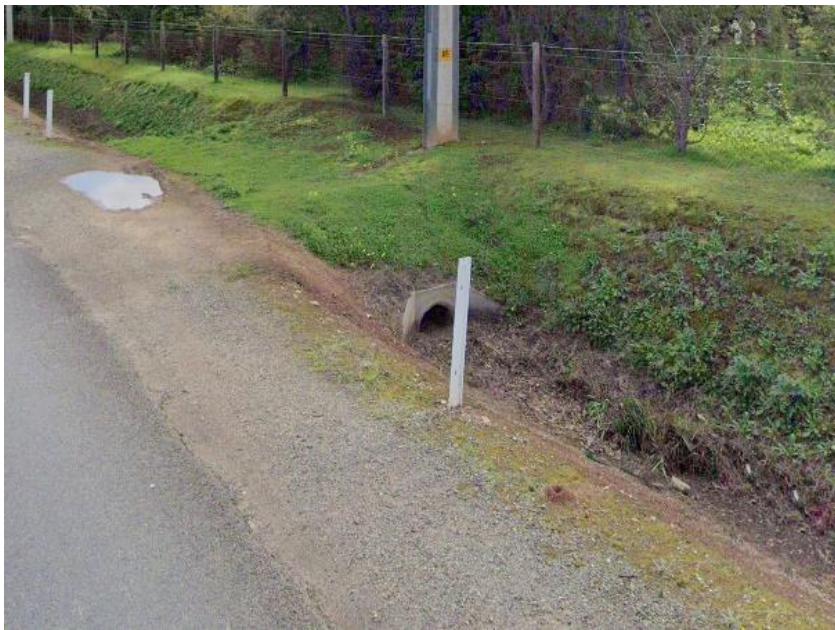
Figure 2.1 Existing Stormwater Infrastructure
