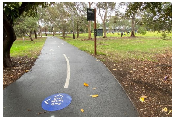
Shared path along Jeffcott Road on the western side of Leroy Oval north of Barton Terrace West
