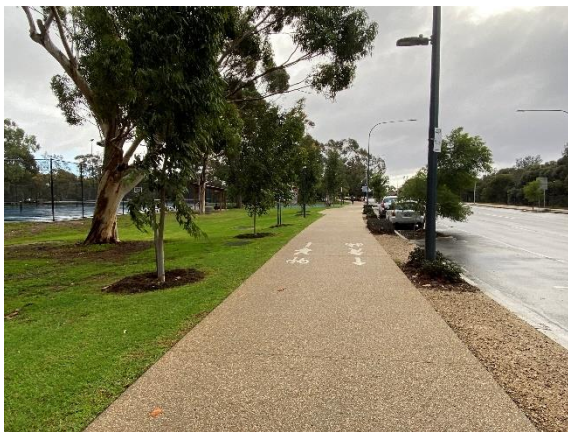
Shared path along the west side of Prospect Road between Barton Terrace West and Fitzroy Terrace
