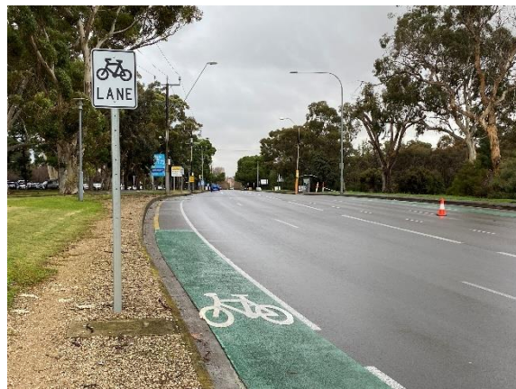
On-road bicycle lane along the west side of Jeffcott Road heading to the entrance of the Aquatic Centre
