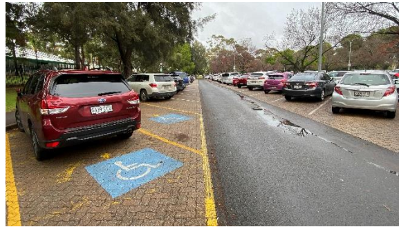
Car park looking south with disabled access spaces
