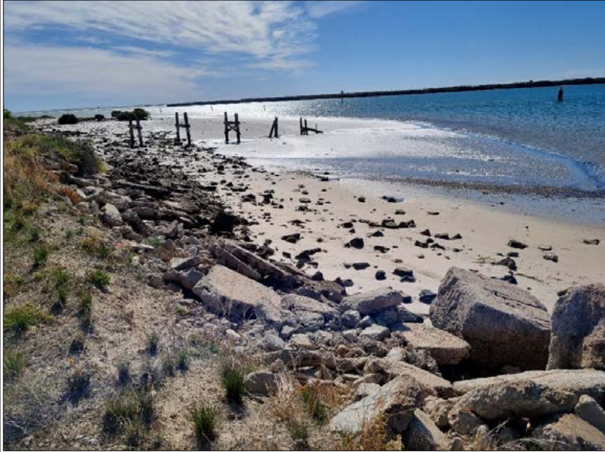
CT A – CONCRETE SLABS AND OTHER FILL ALONG EASTERN BOUNDARY
