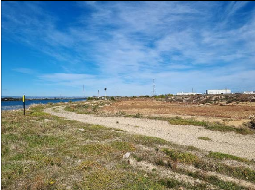
CT A – EASTERN DREDGE POND
