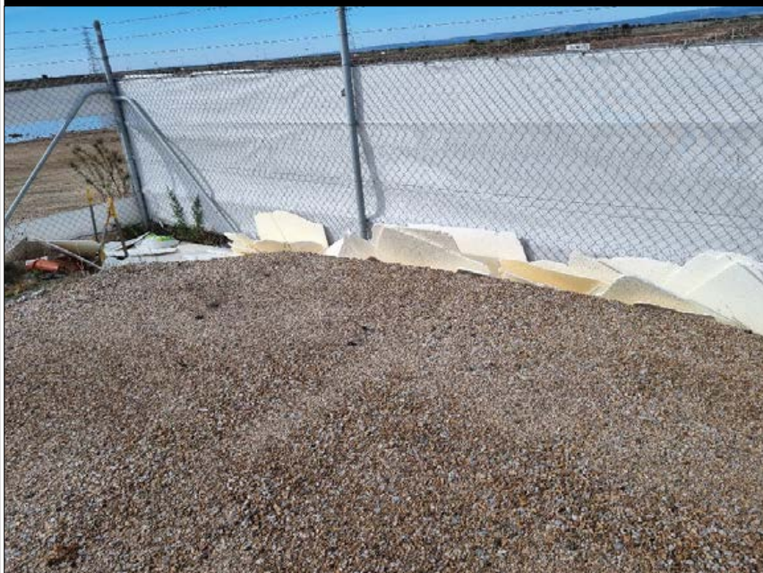
CT L – RUBBISH ALONG FENCE LINE
