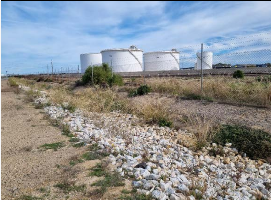
CT L – DRAINAGE SWALE ALONG WESTERN SIDE
