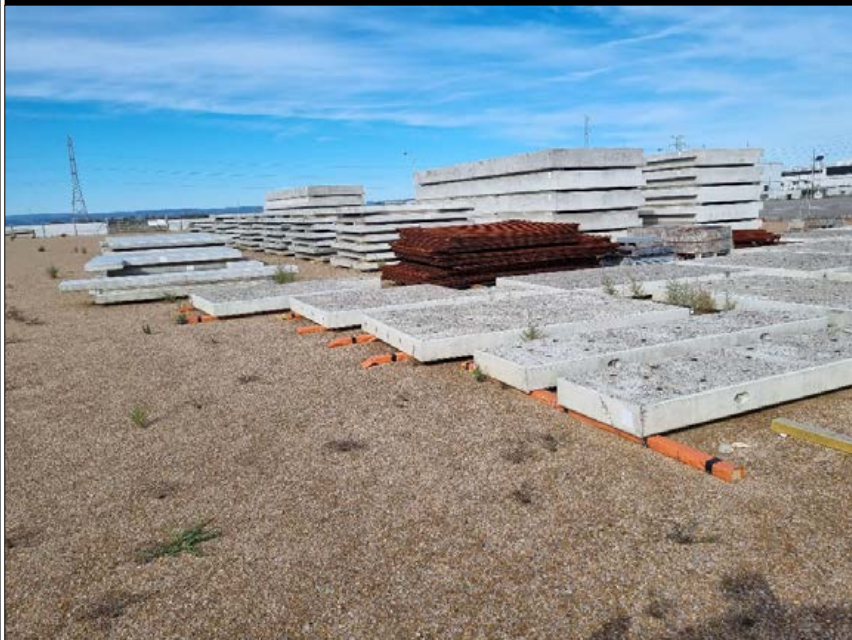
CT O – LAYDOWN AREA WITH PRECAST SLAB AND MATERIALS STORAGE
