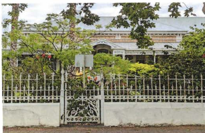
13 Fitzroy Tce Expanded two storey cement slab nursing home approved by the ERD court in the back
