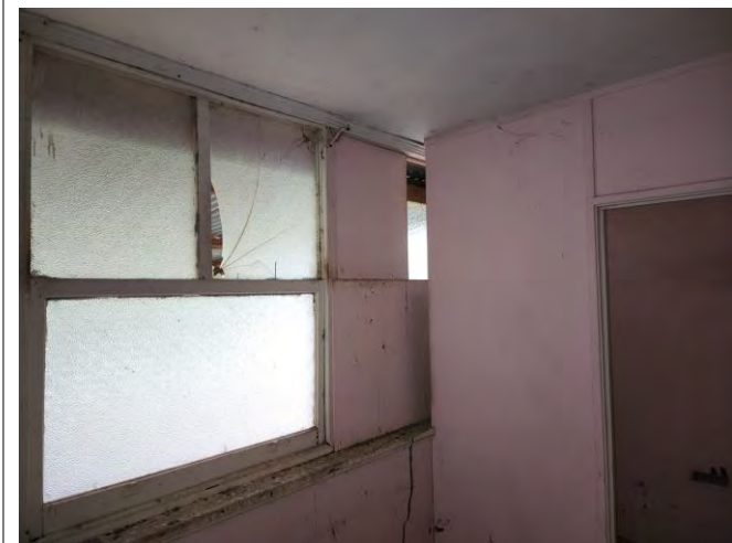
Item 3 – House, infills (internal)
