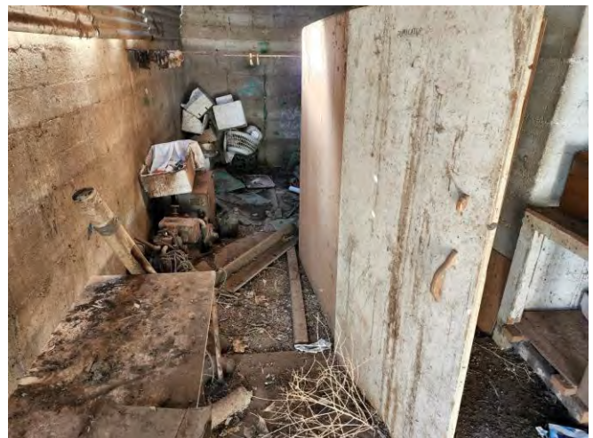
Item 10 – Small Shed, floor (overview)
