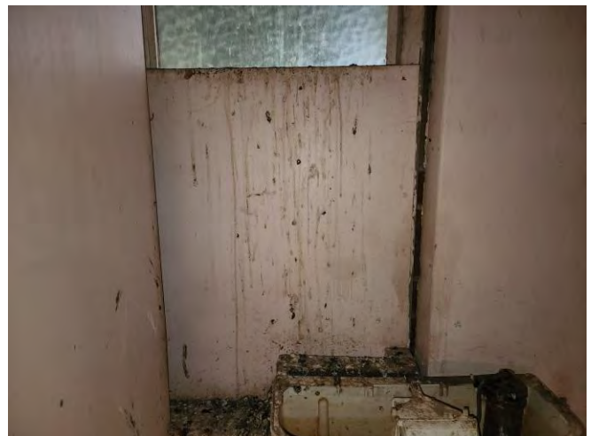
Item 3 – House, infills (internal)
