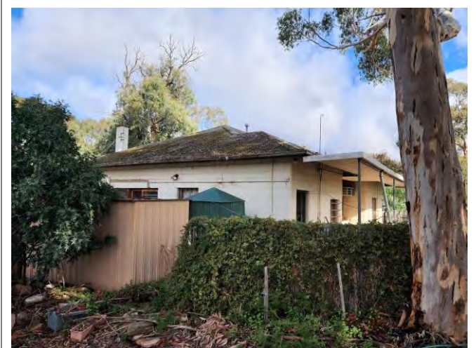
Item 5 – House, roof cladding
