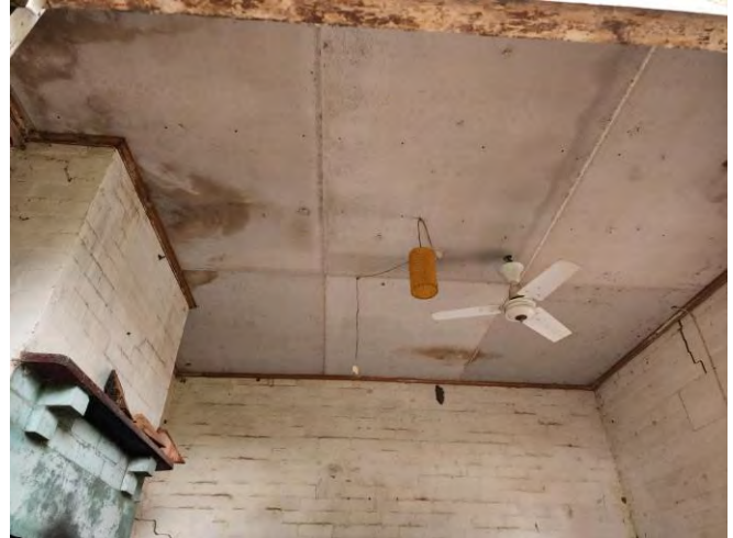
Item 13 – Shearer's Quarters, south room, ceiling
