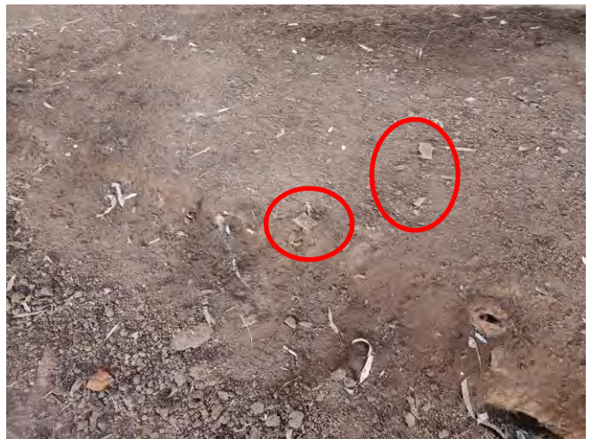
Item 13 – Eastern Chicken Shed – Debris throughout
