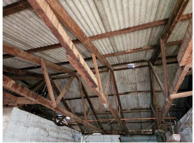
Item 7 – Small Shed roof (internal)
