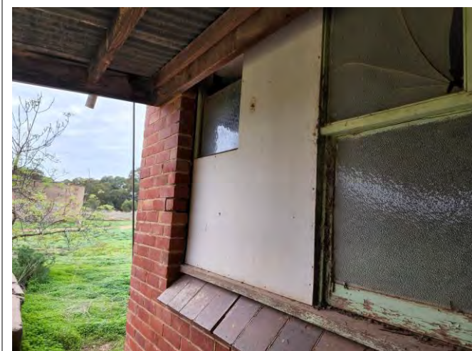
Item 3 – House, infills (external)
