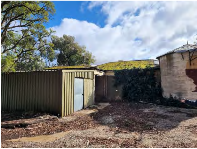
Item 7 – Small Shed roof (external)
