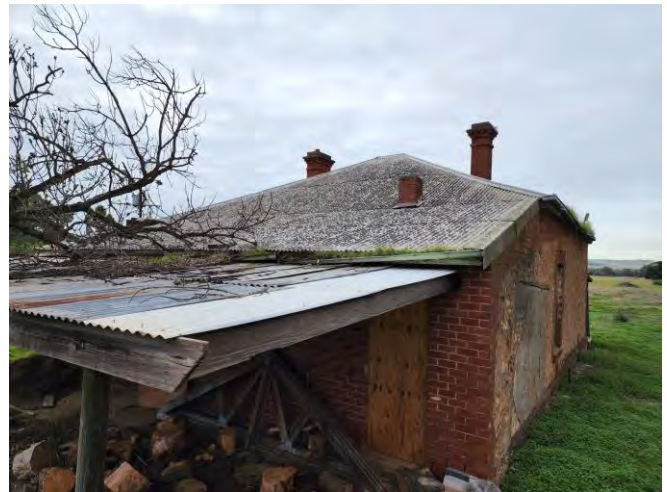
Item 2 – House, roof
