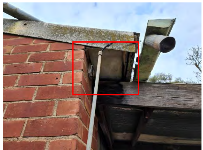
Item 4 – House, eave lining
