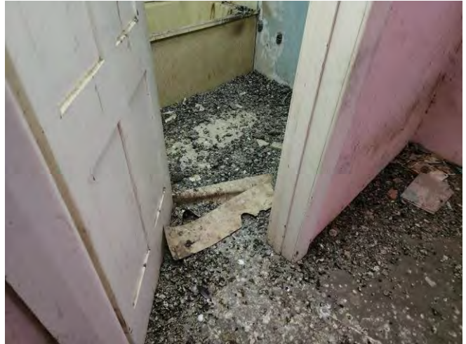
Item 6 – House, bathroom vinyl sheet (No asbestos visible)
