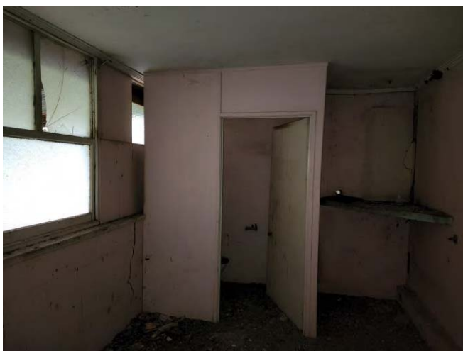
Item 7 – House, toilet walls
