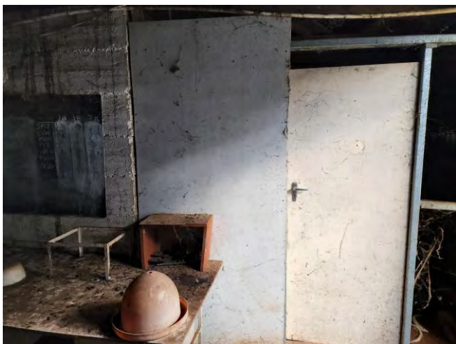
Item 9 – Small Shed, infill panel (No Asbestos Detected)
