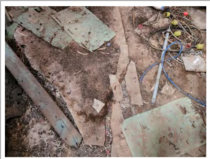
Item 10 – Small Shed, floor (close up)
