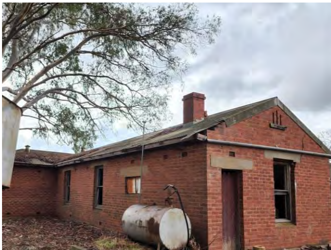
Item 10 – Shearer's Quarters, roof
