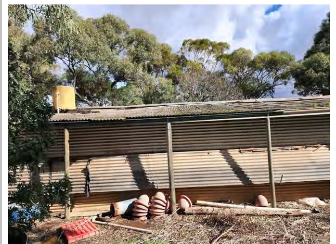
Item 14 & 15 – Central Chicken Shed, roof and low-level walls
