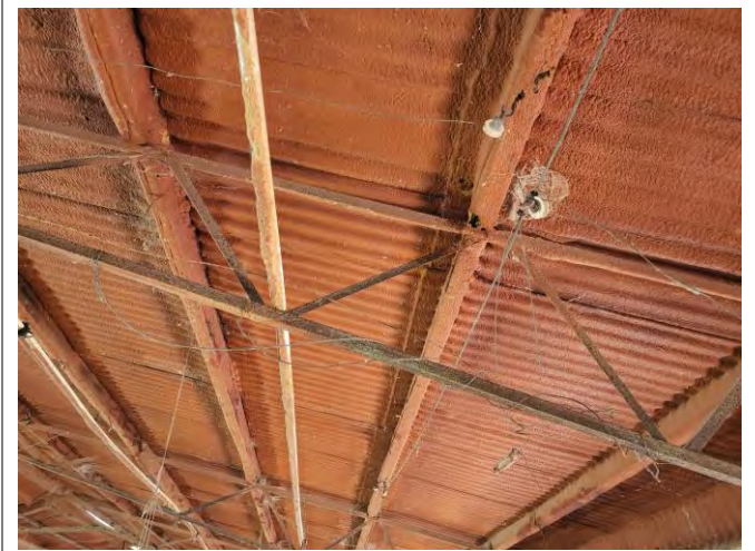
Item 12 – Eastern Chicken Shed, ceiling insulating membrane (No Asbestos Detected)
