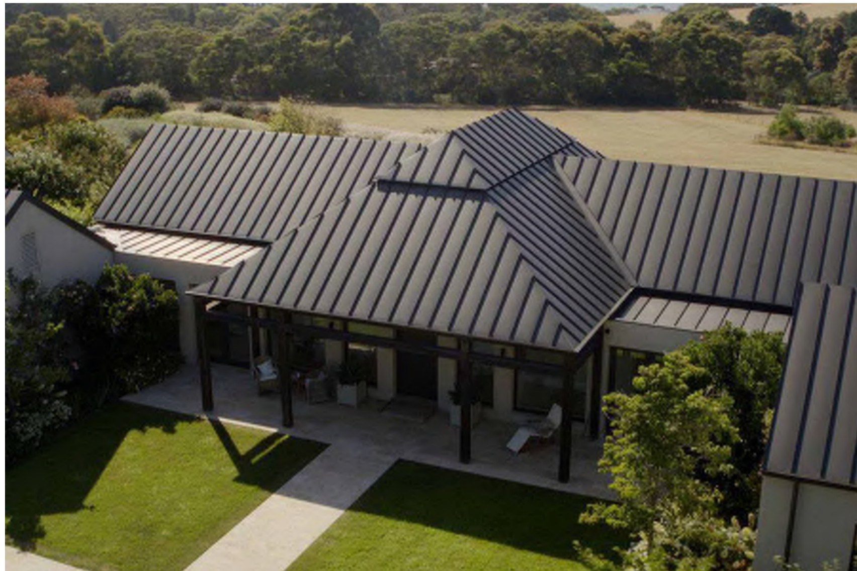
RF-1: STANDINGSEAM METAL ROOF SHEETING - BLACK
