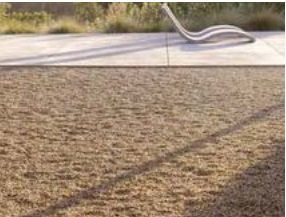
Compacted Sand / Gravel Paving
