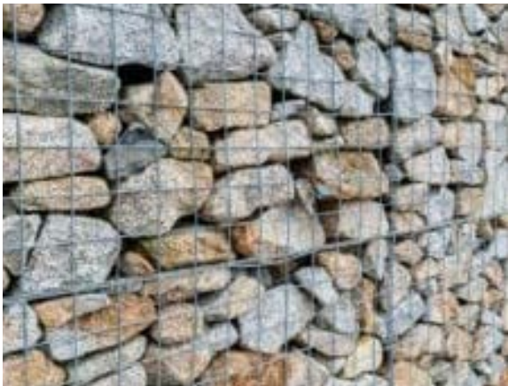
W1 - Gabion Wall - Local Stone
