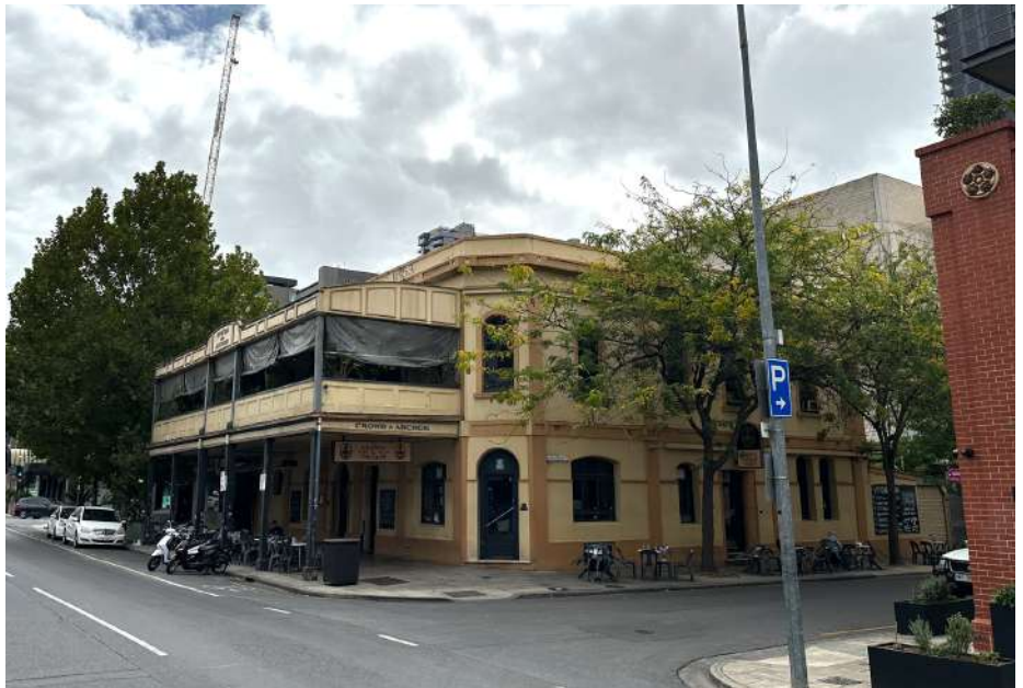
Figure 1: Image of Crown and Anchor Hotel, taken from East (by Author)
