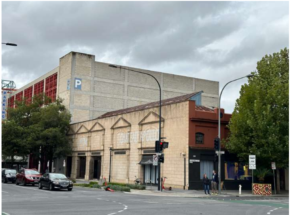
Figure 8: Image of Site 2 along eastern side of Frome Road and along northern side of Grenfell Street (by Author)
