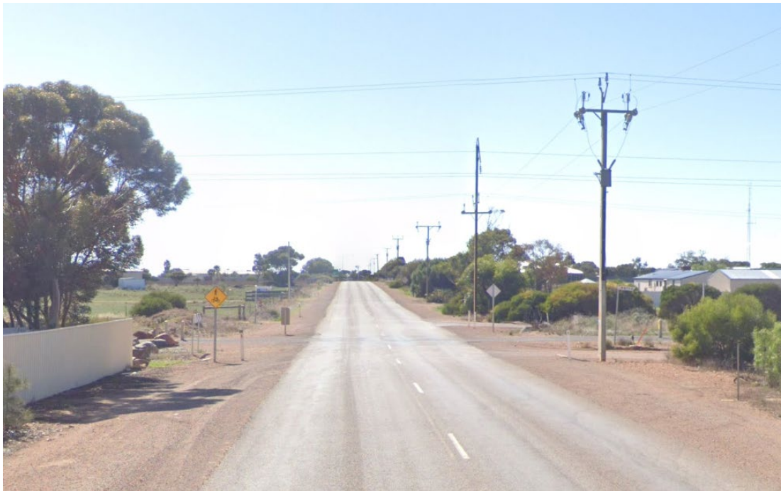
Figure 2 – Existing Rail Trail crossing on Sharples Road
